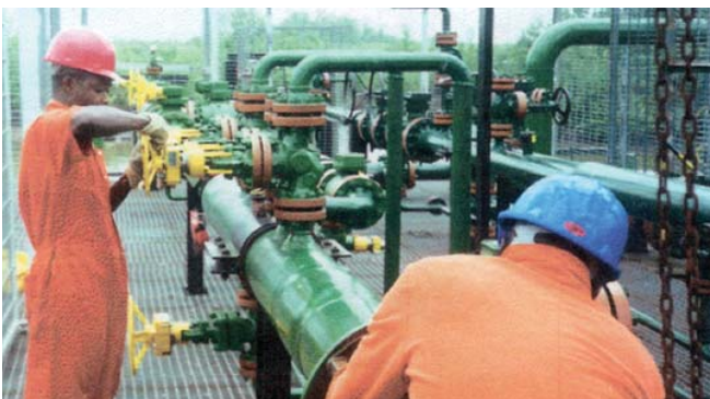
Routine Closure & Valve Interlock maintenance being carried out on site.
